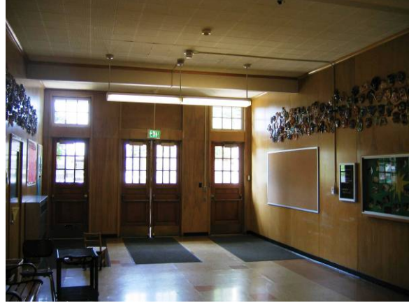
Entry facing south showing newer wood paneling
