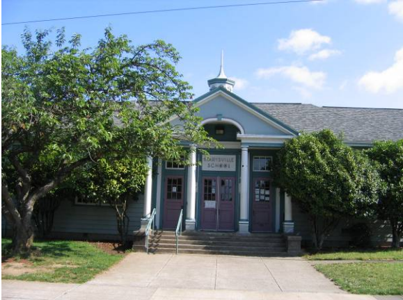
South elevation facing north
