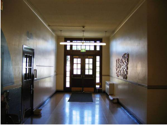
Corridor facing west showing original doors
