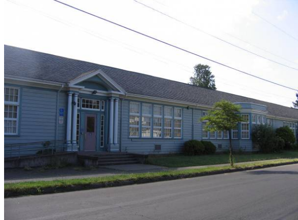
West elevation facing east
