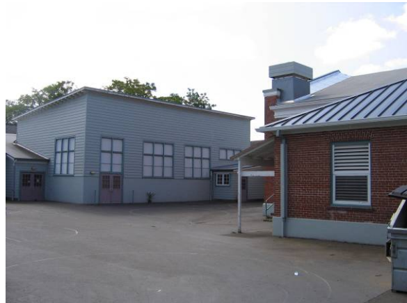
Facing south showing additions on north side
