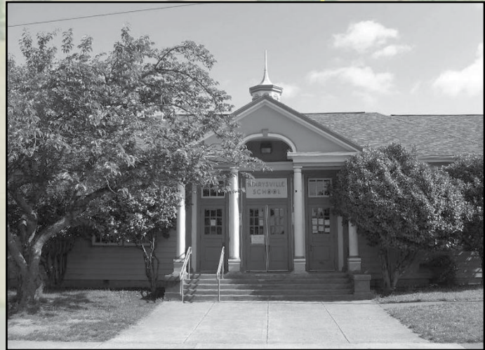
2009 photograph of the front entrance to the Marysville School.
